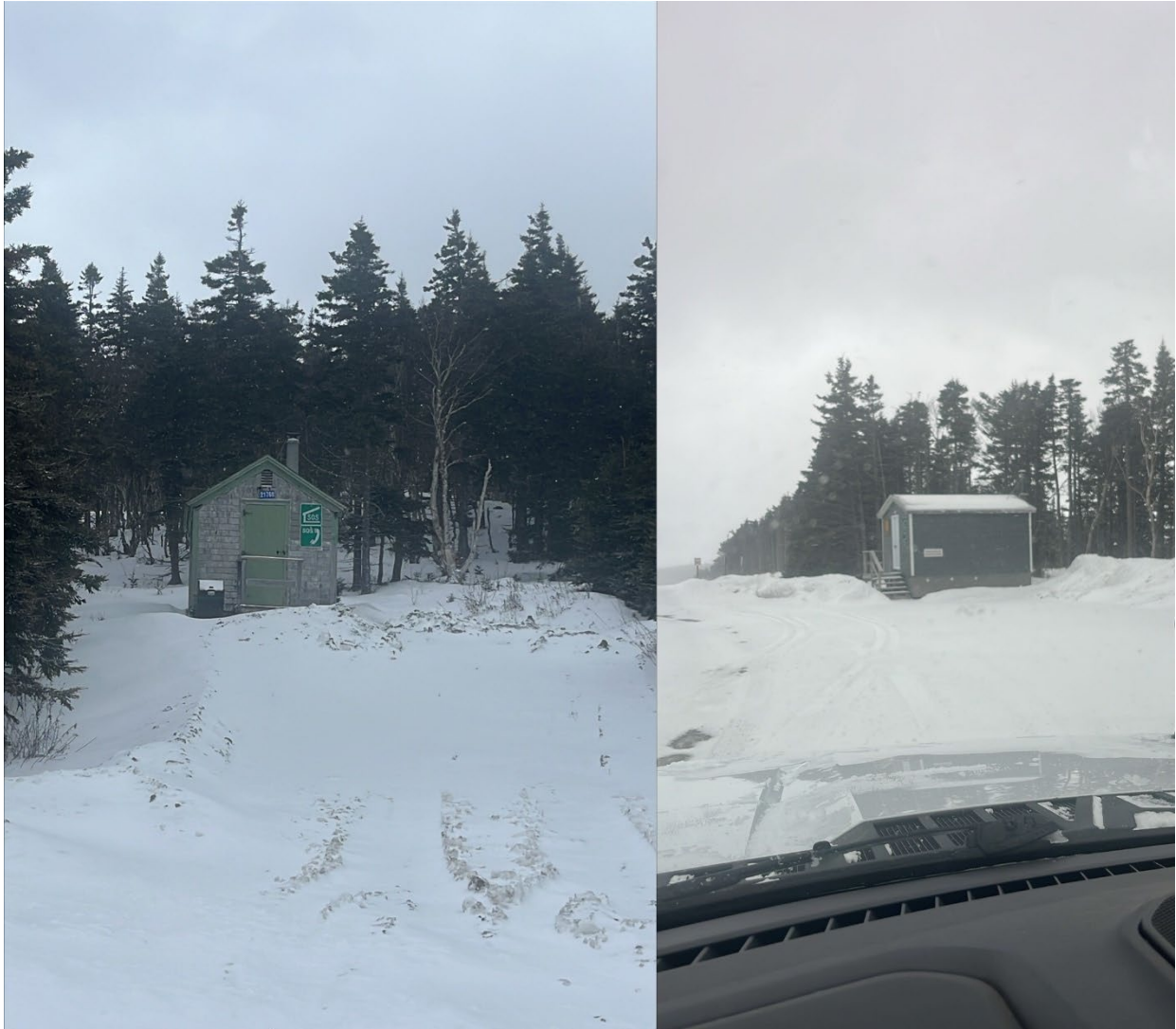
1 Figure 38 – Emergency Huts between North and French Mountain along 85S-401
