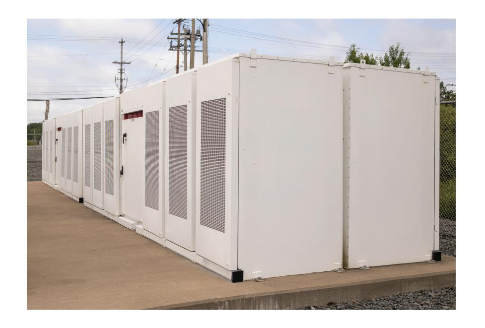
As we move towards a larger portion of electricity on the grid being provided by intermittent sources -such as solar and wind- battery storage technologies such as grid scale batteries will be increasingly important to store excess renewable energy when it is available, and move this supply to when there is not enough capacity to meet demand.
