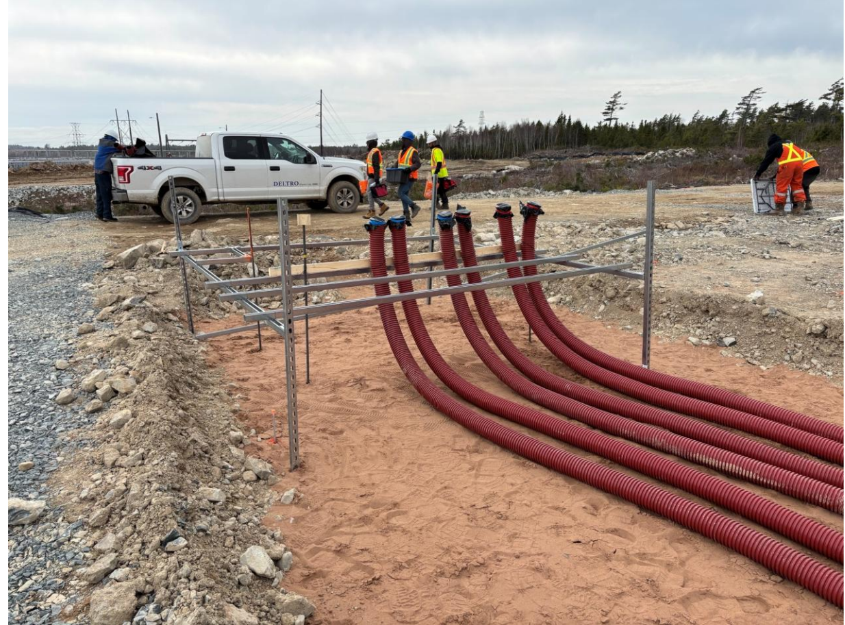
Cable conduit for battery placement
