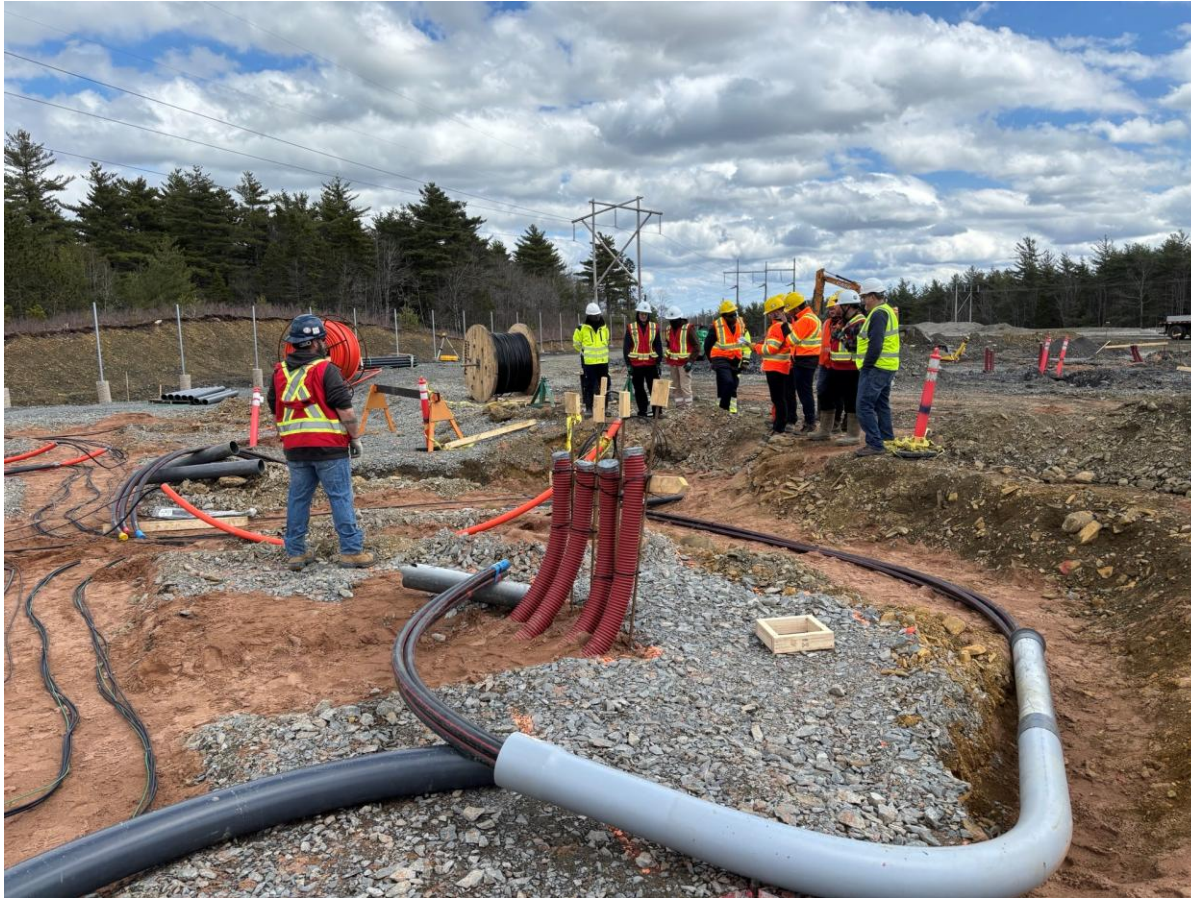
Crews oversee placement of cables and conduit
