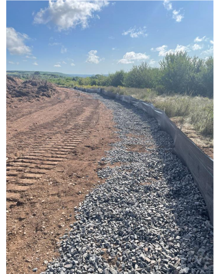
Silt fencing placed to avoid run-off
