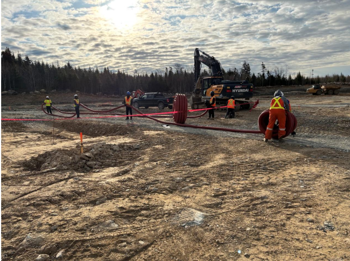
Sub-contractors/ crews place DC cable conduit – April 2025
